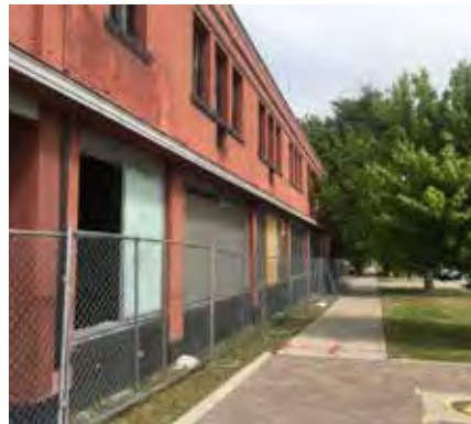
Renovation at North Temple and 600 W
