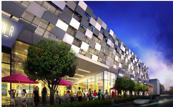
Miami, Florida Parking Structure
